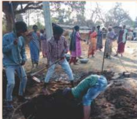
Construction of Soak-pit, Barguttu Village, Ranchi
